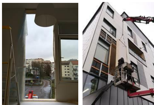
Fig. 4. Installation of the mock-up wall at HSB Living Lab.
