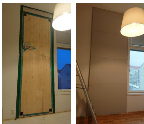
Fig. 5. The completion of the mock-up installation.
