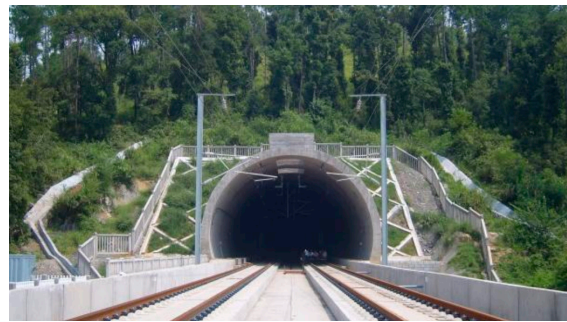
Figure 8. The Pingtu tunnel used for real train experiment.
