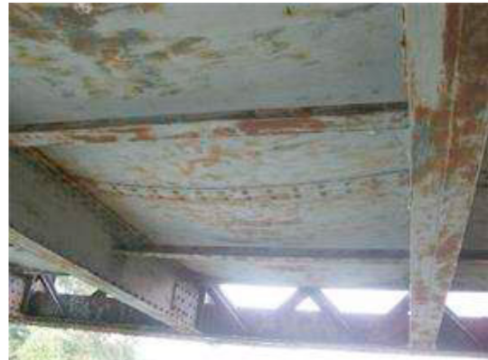
Figure 3 : steel-concrete composite deck (built around 1900)
