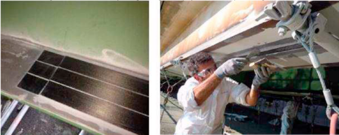
Figure 15 : Implementation of the carbon plates
