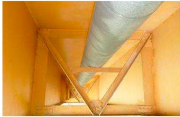
Intermediate beams and bottom flange of composite deck
