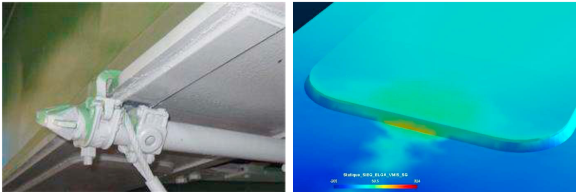
A - View of the ends of the cover plates with the carbon fibers stripes
