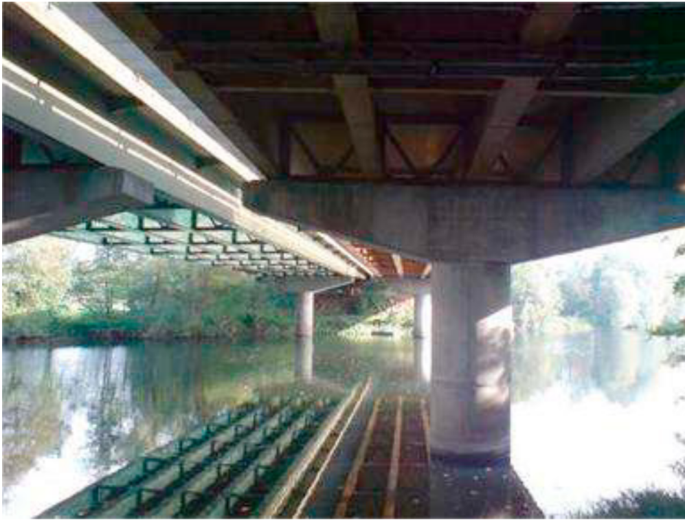
Figure 1 : Sight of the beams of the two independent bridges supporting the highway
