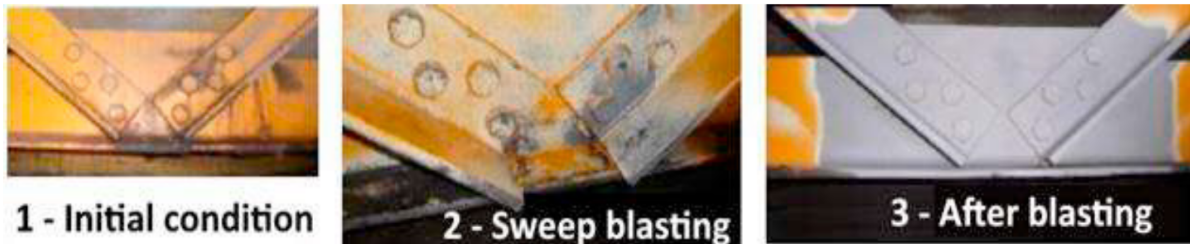
Figure 17 : Intermediate transverse beam at different blasting levels
