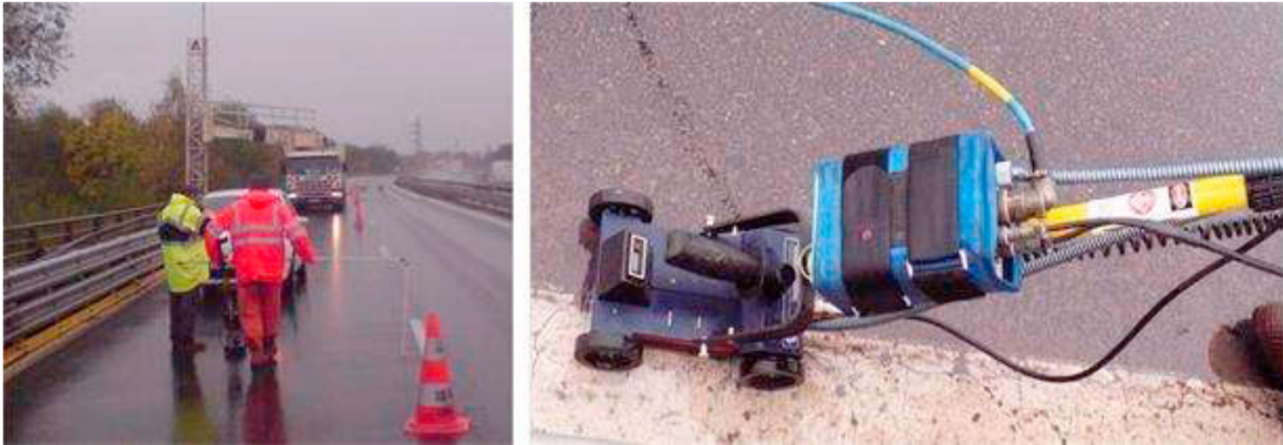
Figure 7 : Radar examination of the composite slab and its waterproofing
