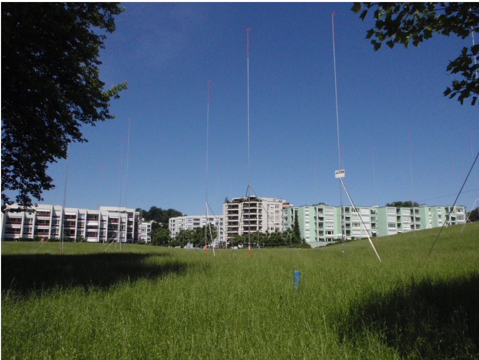
Figure 40. Baugespann. Example from Schönbühlring in Lucerne, Switzerland. (Author: 2011pnm, Source: https://commons.wikimedia.org/wiki/File:Sch%C3%B6nb%C3%BChlring_in_Luzern.jpg )
