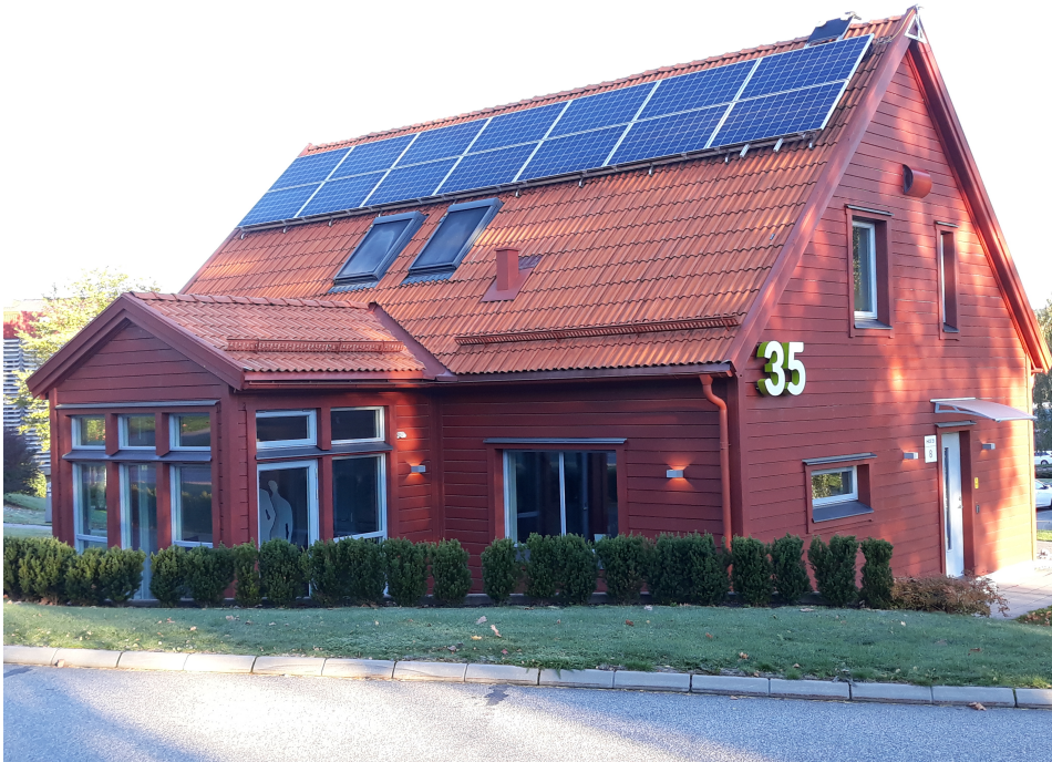
Figure 3.1: RISE Research Villa in Borås, Sweden used for demonstrating the DC system operation with Solar PV, battery storage and DC operated loads.
