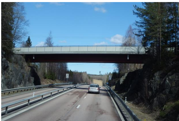
Figure 15. The simply supported road bridge.
