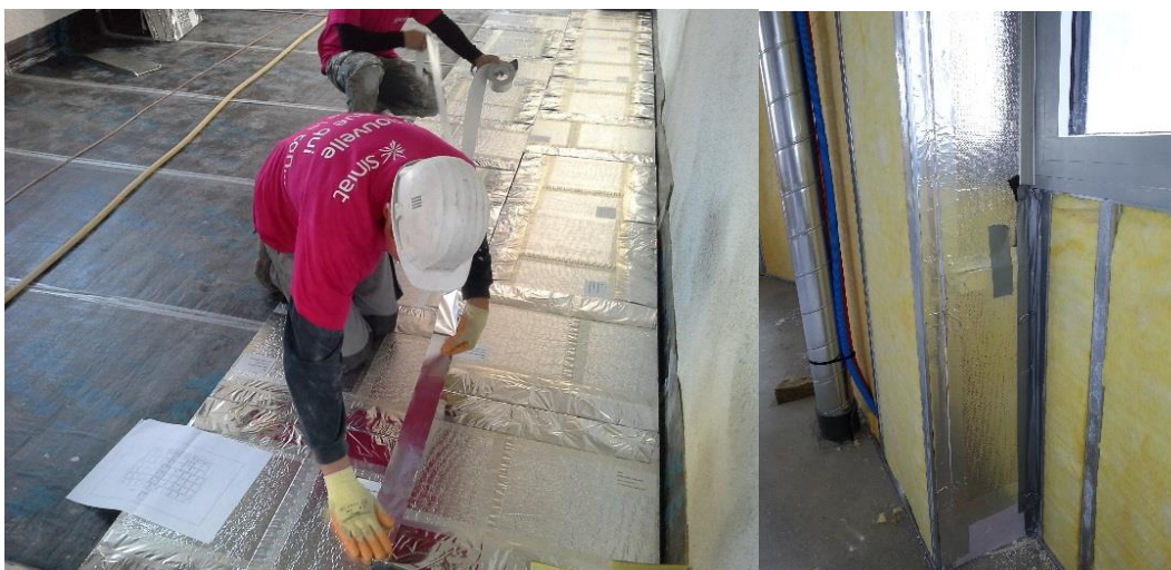
Figure 3-18: Building in Nantes insulated with VIPs in floor and on the interior of the existing walls (Photo: POUGET Consultants).
