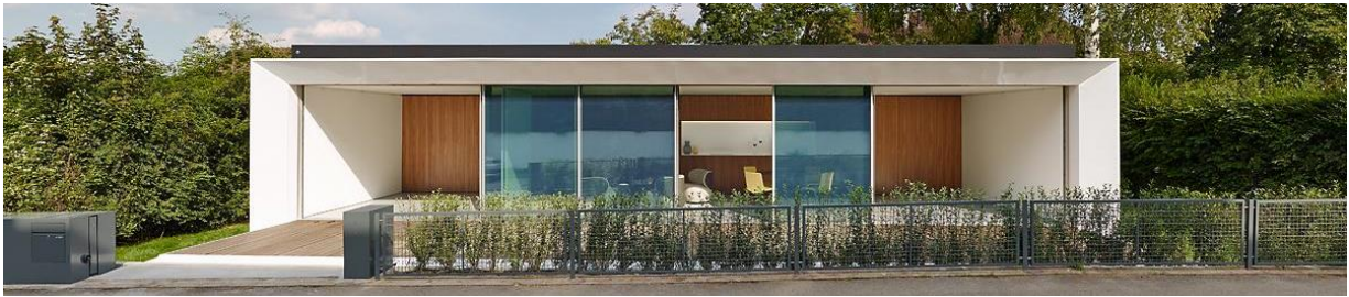
Figure 3-15: House with walls and ceiling containing VIPs [64].
