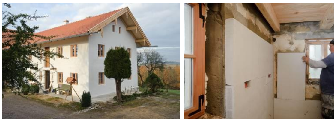
Figure 3-8: Refurbishment of a 150 year old farmhouse [59].
