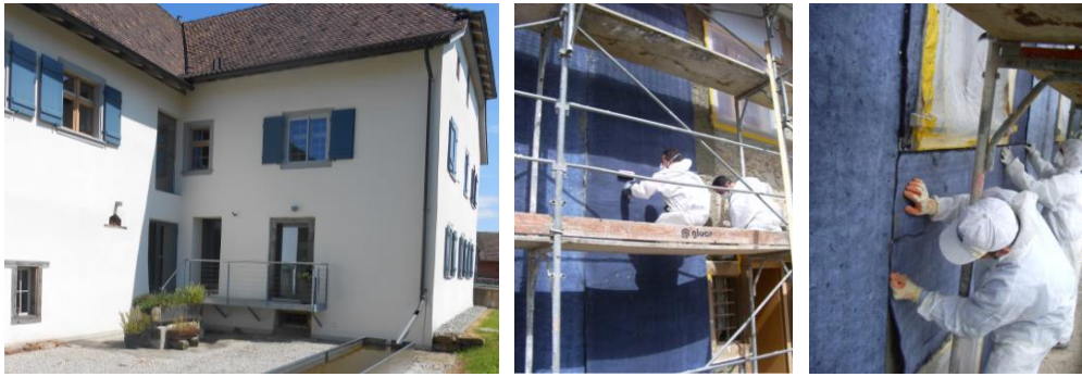
Figure 3-4: Old mill renovated in Oberhallau, Switzerland [54].
