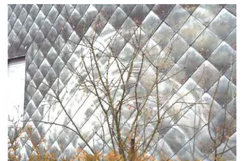
Figure 2.105: Concrete tiles on the weathered surface of which a drawing by wind and scrubbing branches has deposited. Photograph: Thierry Berlemont.
