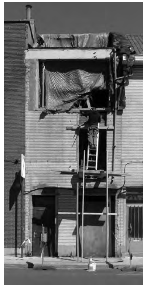
Figure 2.91-94: Front façade of the Research Studiolo, preparing the structure for and charring the wooden cladding, with some help of the former CoMa/ CoIn student and STUDIOLOarchitectuur intern Mirte Van Aalst. Photographs: Joban Liekens.
