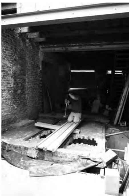
Figure 2.71-73: The discovery of a former cellar and subsequent elaboration of a formwork of roughly sawn wooden planking to pour concrete walls with wood imprint. Photographs: Johan Liekens.
