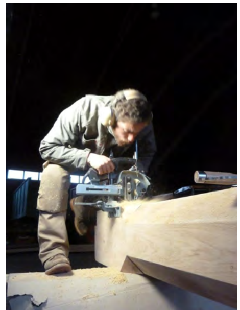
Figure 0.5: Seppe Geuens of Compagnons preparing the wooden center pillar of a medieval gateway. Photograph: Compagnons .
