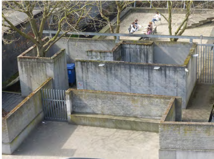
Figure 2.55: Original concrete bench with cinderblock wall added on top, enclosing the former public garden. Photograph: Johan Liekens.
