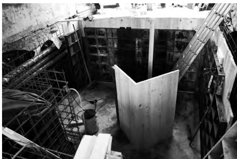
Figure 2.71-73: The discovery of a former cellar and subsequent elaboration of a formwork of roughly sawn wooden planking to pour concrete walls with wood imprint. Photographs: Johan Liekens.
