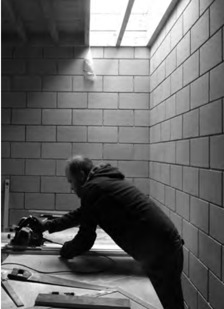
Figure 2.81-84: Creating formwork and casting concrete for the corner object, imitating the back corner and cinderblock patterning of the Research Studiolo's walled contour, to be subsequently displaced in the public terrain, positioned in a receding angle of the former public bench. Photographs, design and execution: Joban Liekens.
