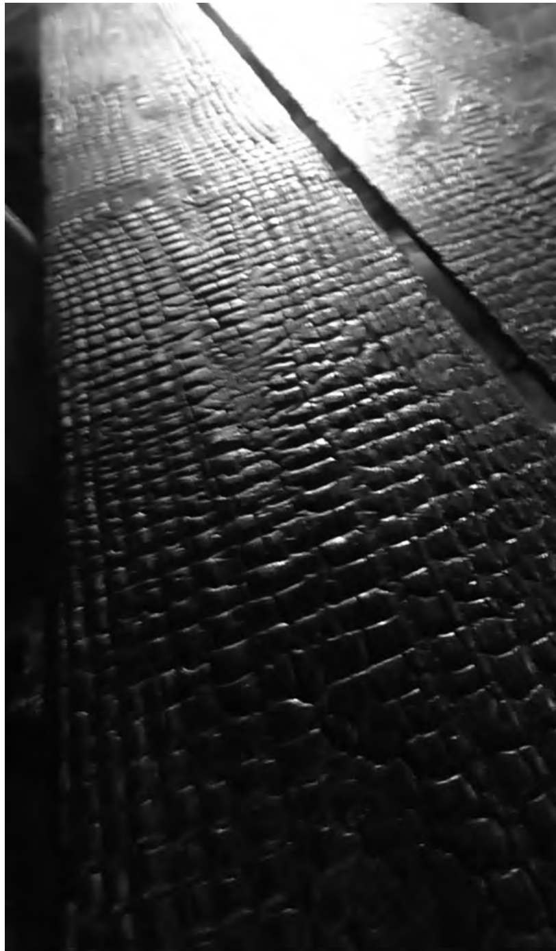
Figure 2.91-94: Front façade of the Research Studiolo, preparing the structure for and charring the wooden cladding, with some help of the former CoMa/ CoIn student and STUDIOLOarchitectuur intern Mirte Van Aalst. Photographs: Joban Liekens.
