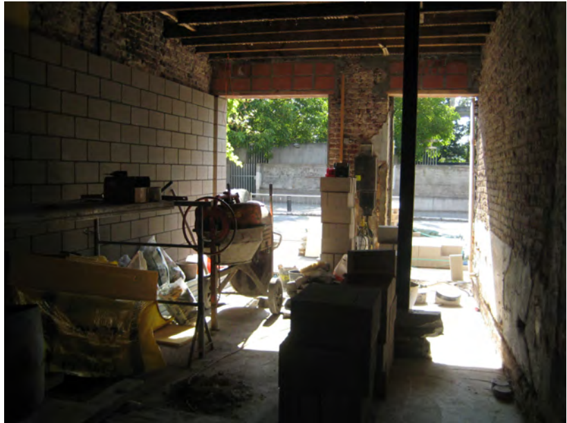
Figure 2.65: Clearing the ground floor of the studiolo's shell. Photograph: Johan Liekens.
