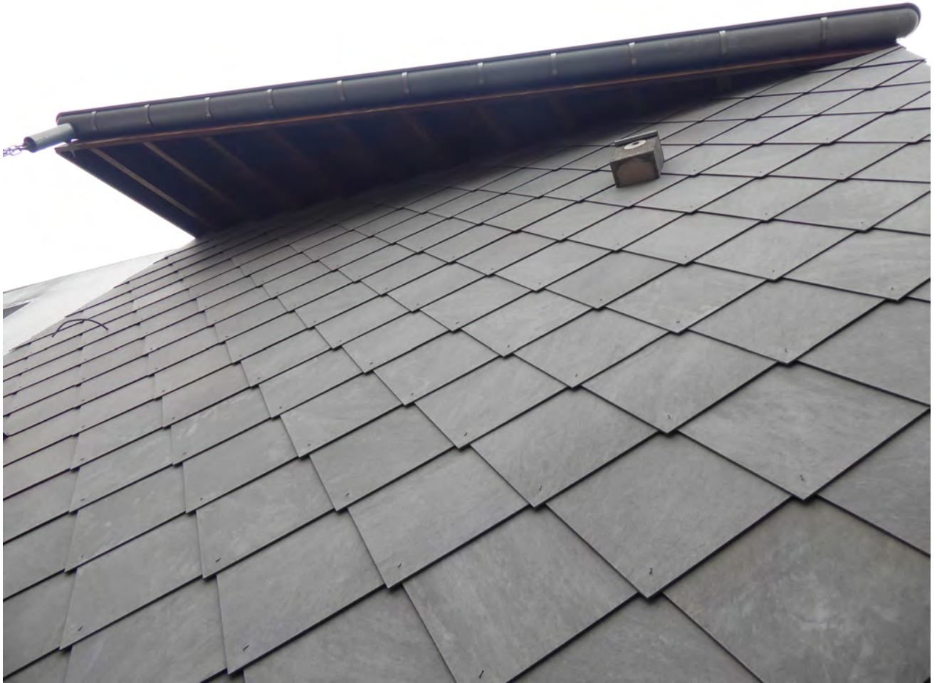
Figure 2.104: The Research Studiolo's rear façade, detailed as a scaled version of the nesting stones it contains. Photograph, design and execution: Johan Liekens.
