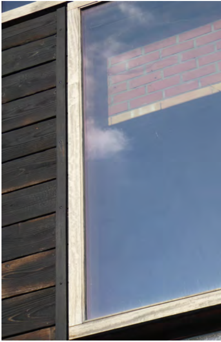
Figure 2.95: Front façade's first-floor window, with wooden block frame following the typology of the neighboring factory houses, while the masonry structure in the depth of the window accords with the contemporary program of the Research Studiolo itself. Photograph: Johan Liekens.
