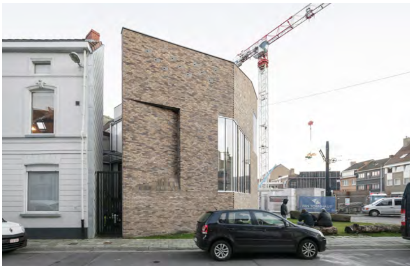
Figure 2.20: Narrow vertical breach separating the brickwork scale from the neighboring building. Photograph: Stijn Bollaert.
