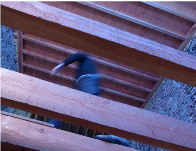
Figure 2.74-75: The sunken surface of the private studiolo with receding alcove (below right) and the open cinderblock contour (above), concrete with an imprint of roughly sawn wooden planking, which was re-used in turn for the ceiling above the sunken surface. Photographs, design and execution: Johan Liekens.
