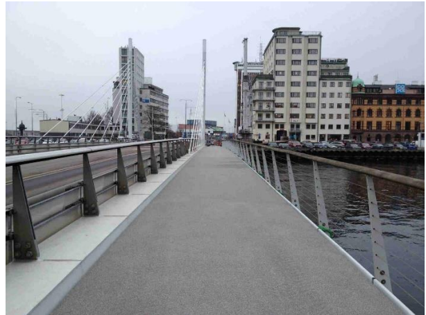
Figure 8. FRP panels installed on sidewalks, Photo courtesy of Per Andersson
