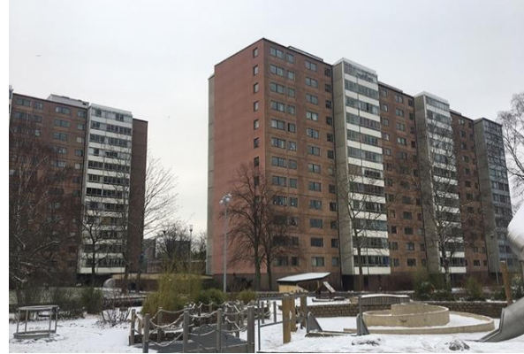
Figure 3. Generic picture of the buildings in Case B. Photo: Authors
