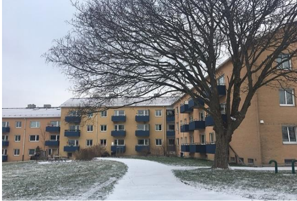
Figure 2. Generic picture of the buildings in Case A. Photo: Authors
