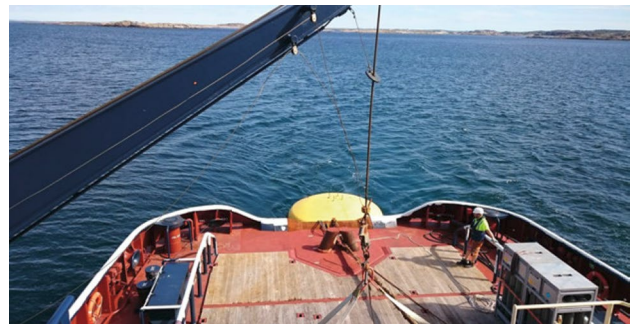
Fig. 4 Simultaneous installation of L12D with its buoy [36]
