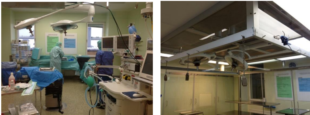
Figure 2.6 Operating room with dilution mixing air (left). Operating room with vertical unidirectional airflow (right).
