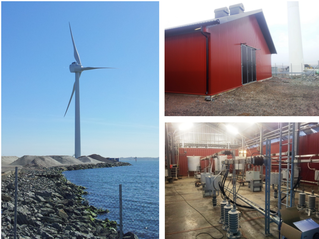
Figure 3. Gothenburg test facility, comprising the 4.1 MW FPC “Big Glenn” wind turbine. The facility houses the back-to-back HVDC station and coupling inductor (back) and AC filters (front).
