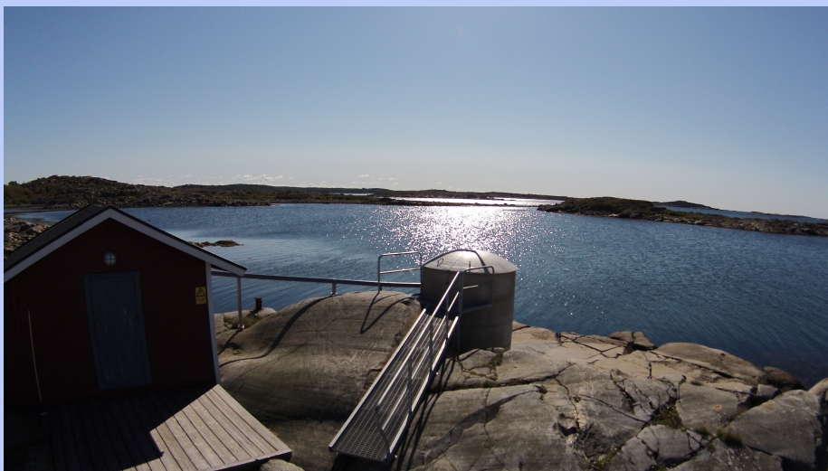
Figure 1. The tide gauge station.
