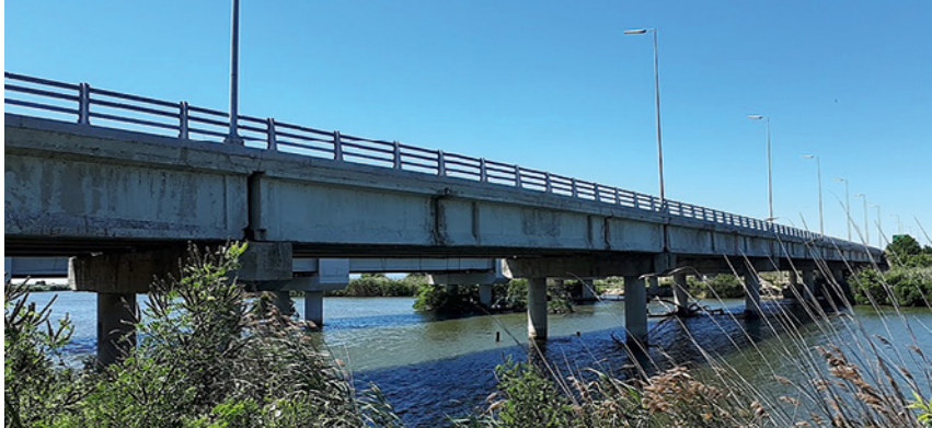
Figure 1. The Strimonas Bridge (Panetsos, 2017)
