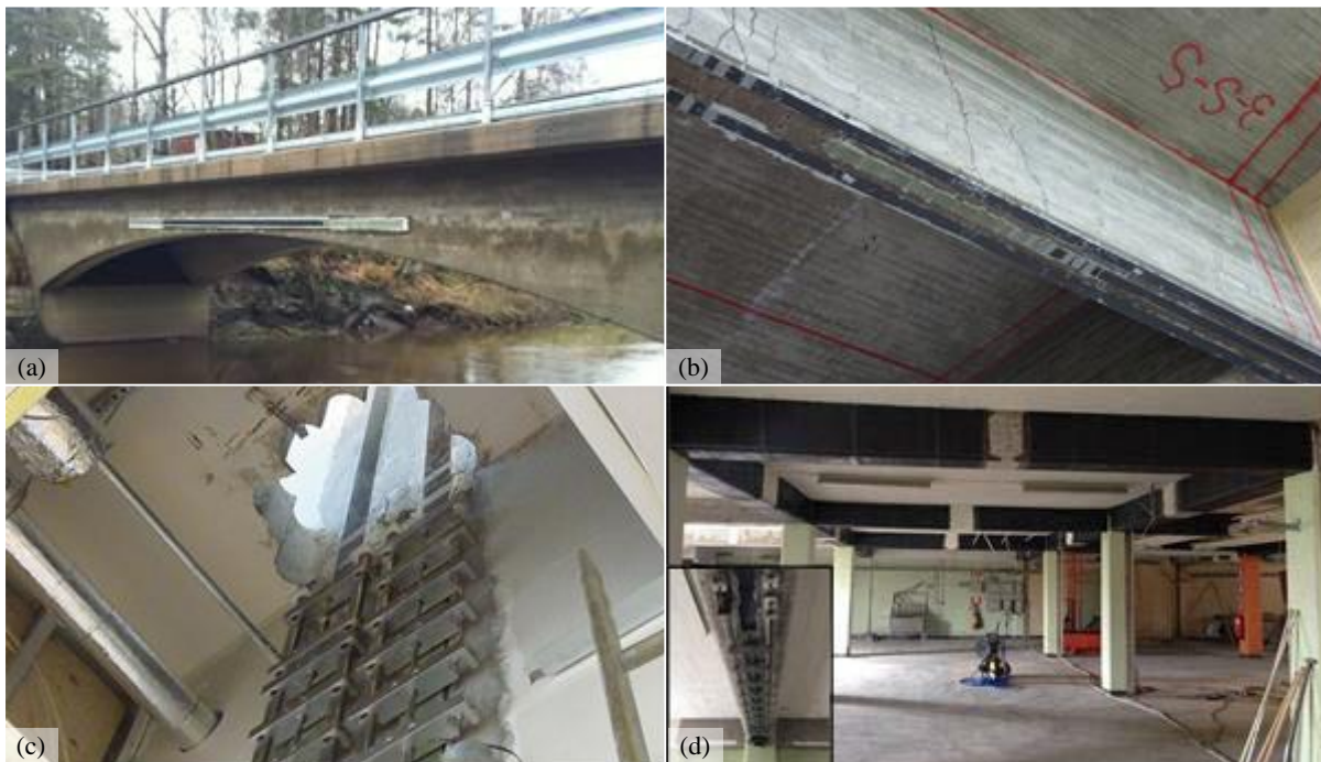
Figure 2.4 Field applications of the stepwise prestressing method (Haghani and Al-Emrani 2016): (a) concrete bridge over Nossan river in Sweden strengthened with one CFRP laminate on each girder prestressed with a force up to 100 kN; (b) concrete bridge located in Kiruna, Sweden strengthened with three prestressed CFRP laminates on one of the girders with a prestressing force of 110 kN per laminate; (c) strengthening of concrete wall segments in a hotel building in Umeå, Sweden using four prestressed CFRP laminates; (d) strengthening of an archive building in Arboga, Sweden with pre-stressed CFRP laminates
