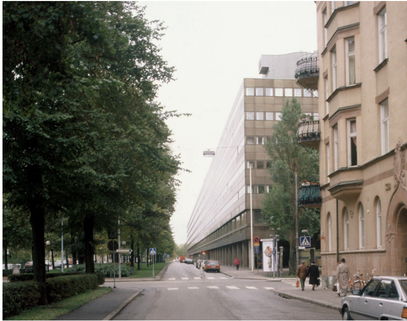
Figure 1. The 346 m long main façade of Garnisonen. Photo by Claes Caldenby.
