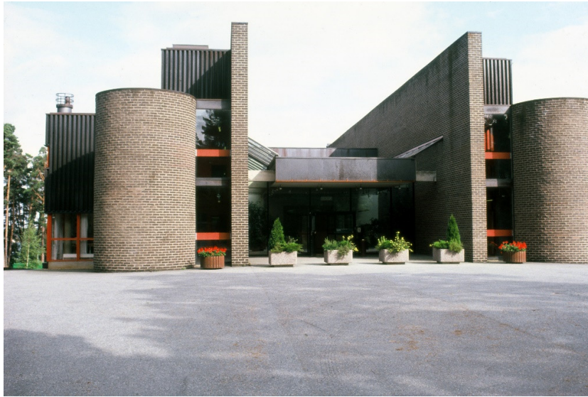
Figure 5. Entrance façade of IBM with staircase towers and a basilica structure with higher auditoriums flanked by two-storey aisles. Photo by Claes Caldenby.
