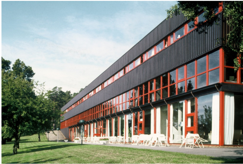
Figure 7. Long side of IBM with restaurant on ground floor, seminar rooms above and hotel rooms on top. Photo by Claes Caldenby.
