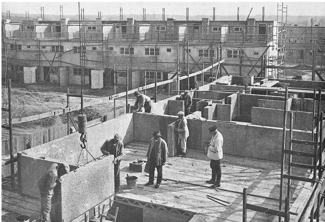
Figure 3. Ernst May: “Frankfurter Montageverfahren” (‘Frankfurt assembly method’). Photo from Das Neue Frankfurt , 1926/1927/2, title.
