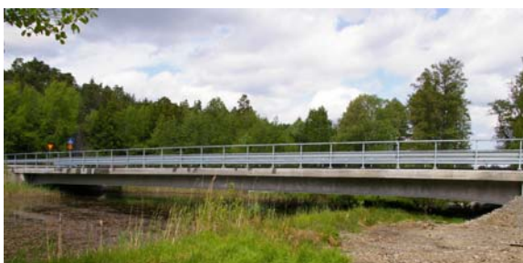
Figure 3: Steel-concrete composite bridge investigated (source: NCC).
