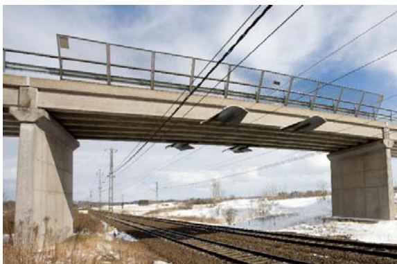
Figure 2: Concrete beam bridge investigated (source: NCC).
