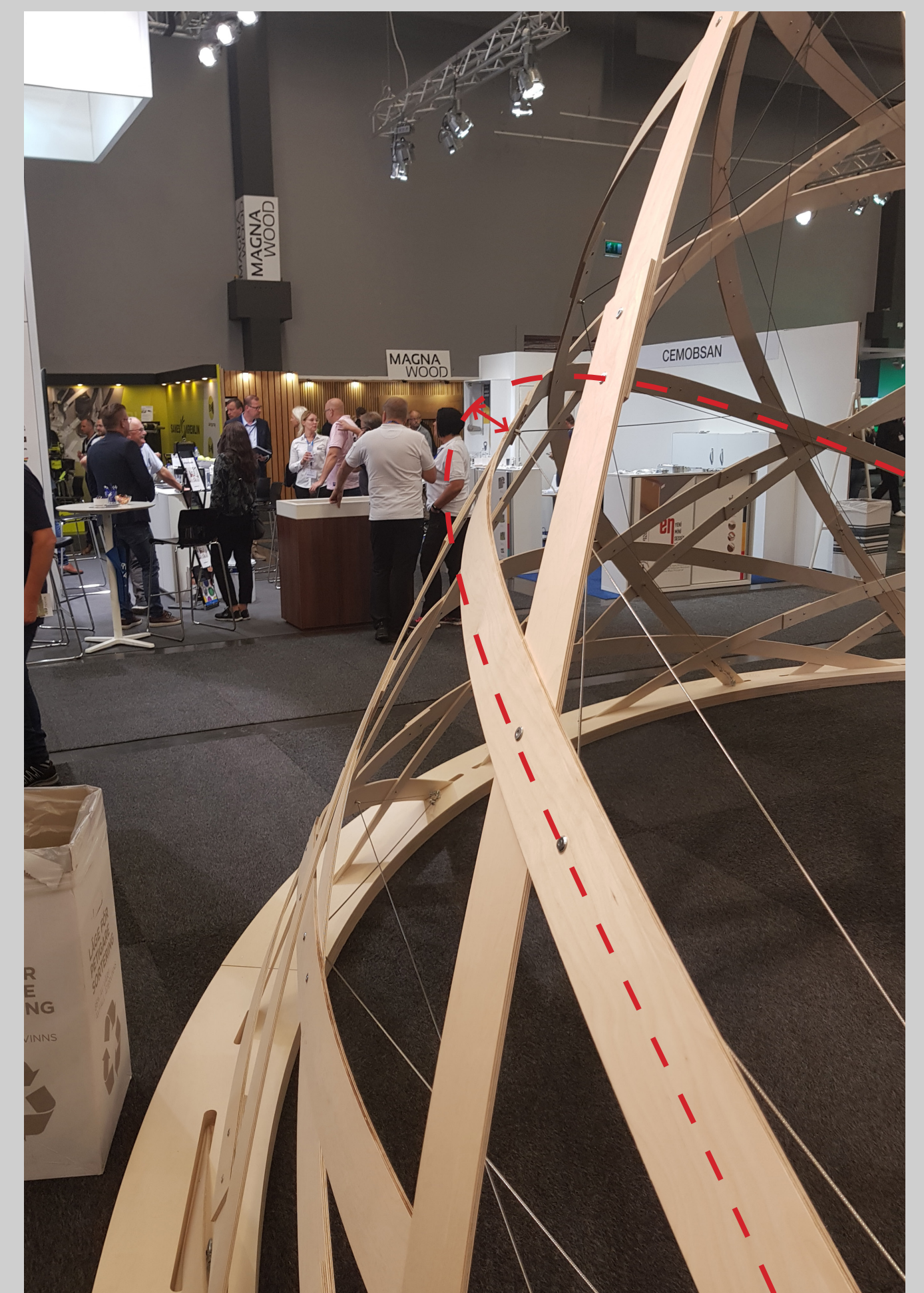
Figure 5: Lath curvature effected by pre-stress.
