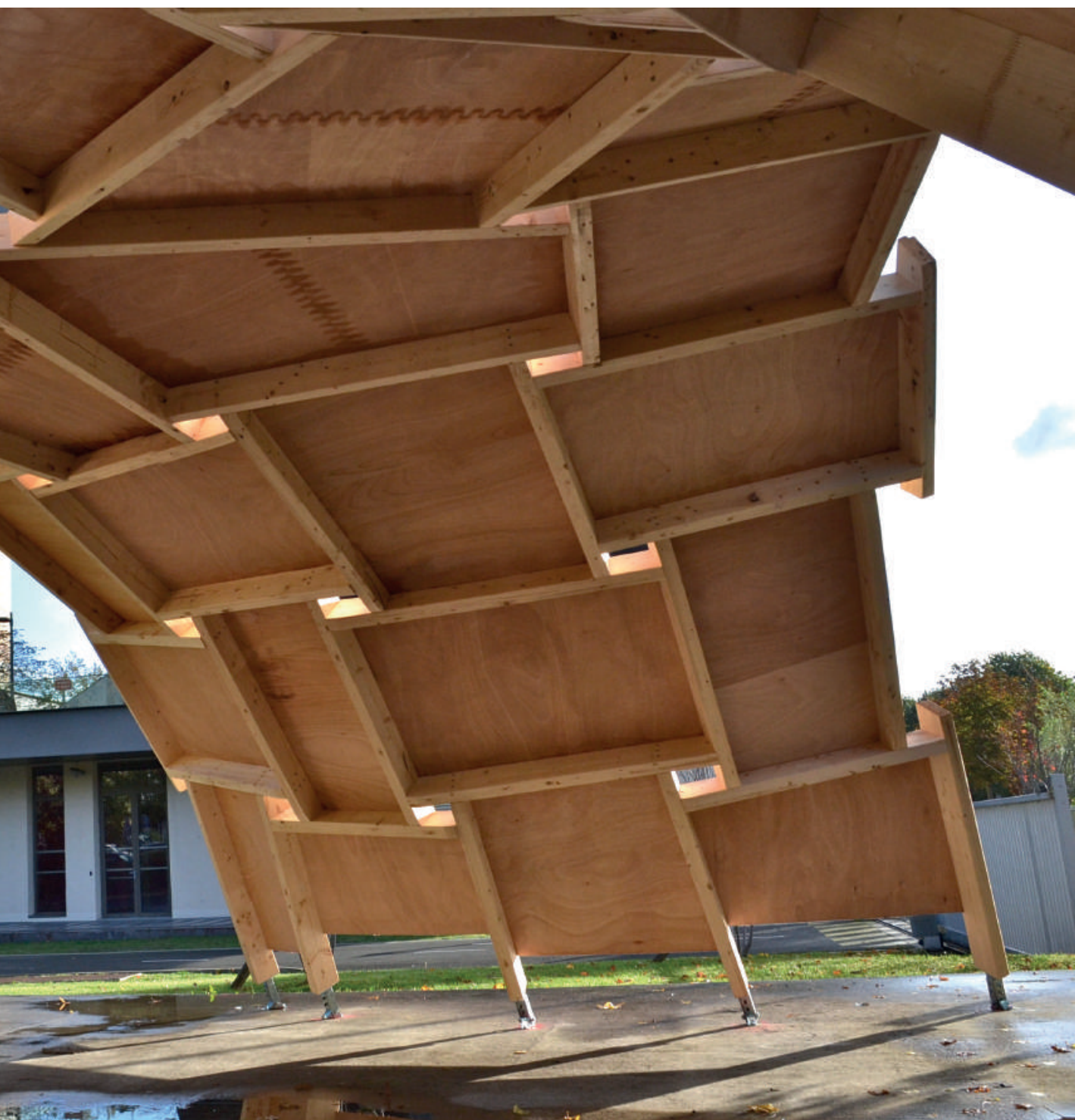
Figure 13: A view of the completed pavilion.
