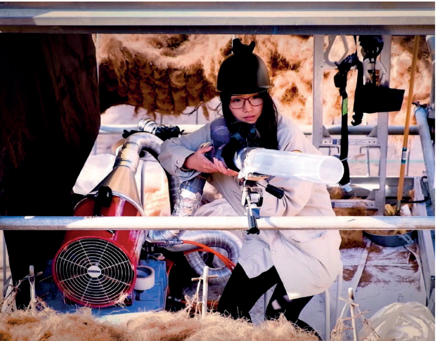
Figure 9: Acoustically guided aiming and shooting process of the pavilion installation using the bazooka projectile tool located in one of the shooting points.
