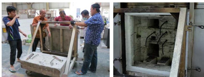
Figure 22 Sample installation and furnace at (PUSKIM, 2015)
