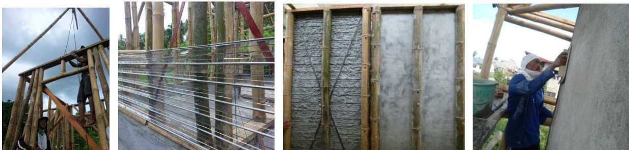
Pictures 1-4. Construction System using prefabricated bamboo frames and mortar coating
