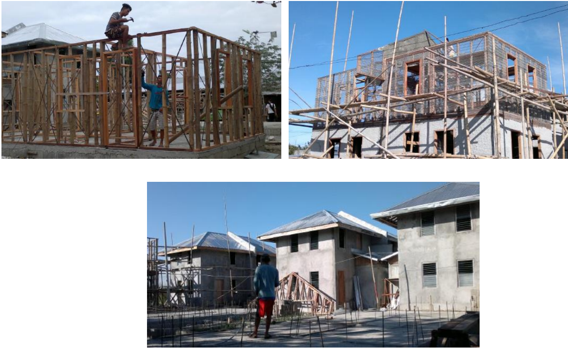
Pictures 5-7. Construction of ten two-story duplex houses, Iloilo City, March 2015 [11]
