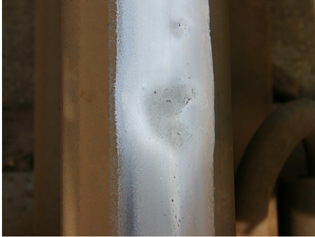
Figure 1.1: A typical squat-like defect found in Stockholm, Sweden. Two distinct lobes are clearly visible. Also note the V-shaped surface breaking crack and the slight widening of the running band.
