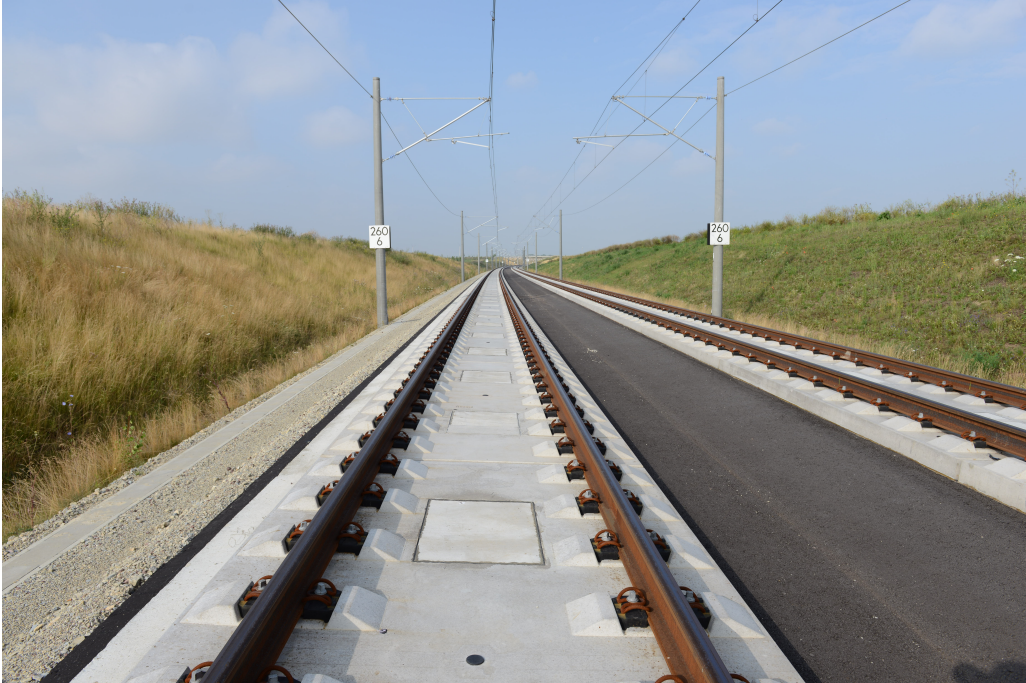
Figure 2.4: Final STA system ready for traffic. From STA [5].
