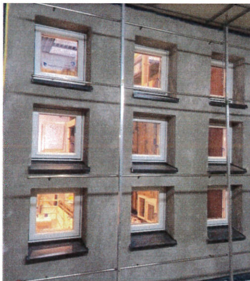
Fig. 4 Front façade of wall 3 installed in the rain chamber
